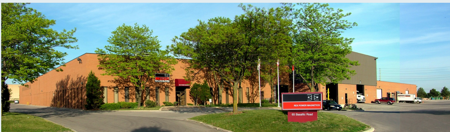
Our 145 000 sq. ft. design, manufacturing, and customer service facility in Toronto, Ontario
